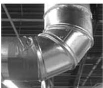
**DO NOT** install sensing tube in an elbow.
